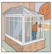
Next the roof is installed. The installer will glaze the roof & fit the sealed glass units to the side frames.
