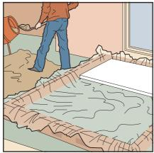
With the foundations laid and the wall constructed to finished floor level, the installer will now prepare the floor slab.
