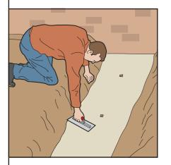
The installer will prepare the site, dig the foundations, install necessary drainage and lay a concrete foundation.
